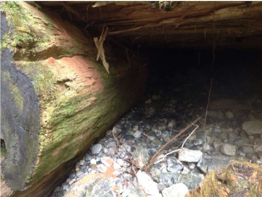
Right Bank Abutment when facing downstream
