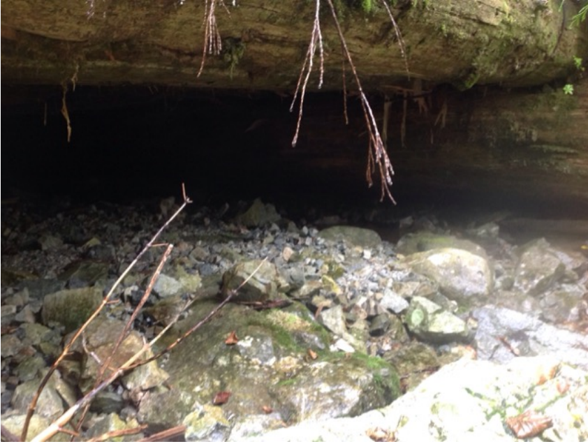
Left Bank Abutment when facing downstream
